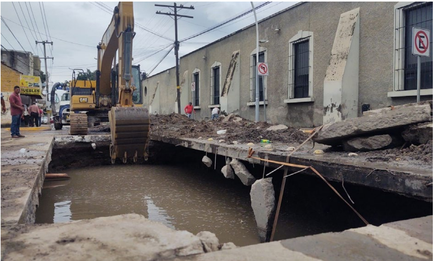
Figure 1.3: Failure of water drainage and the process of erosion in the streets of Tepic, near Sugarmil Source: Antonio Echevarría García vía Facebook.
